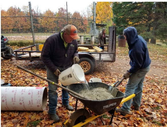
Left: Dan Palosaari and Will Hagelthorn mixing Quikrete; Right: Pete Torola finishing the surface before applying the pattern and adding J-bolts
