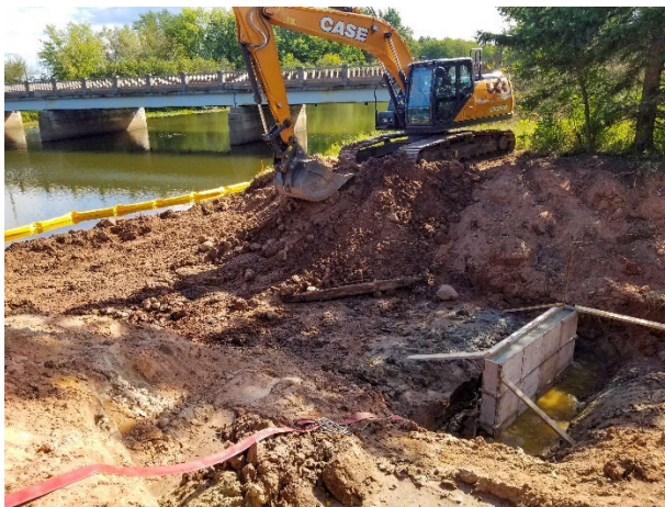
Excavation of the Sturgeon River bank with the headwall already poured.
