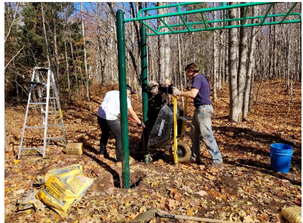
Installing the horizontal ladder
