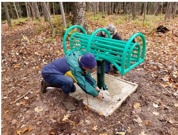
Bill Binroth and Dennis Karvakko tightening down the nuts on the J-bolts
