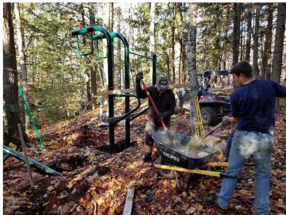
Through a combination of 2 x 4s nailed to trees and twine, Pete found a way to get this station level.
