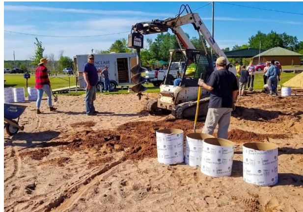
Sleeves for the holes were cut by these MTU athletes and then placed in the drilled holes
