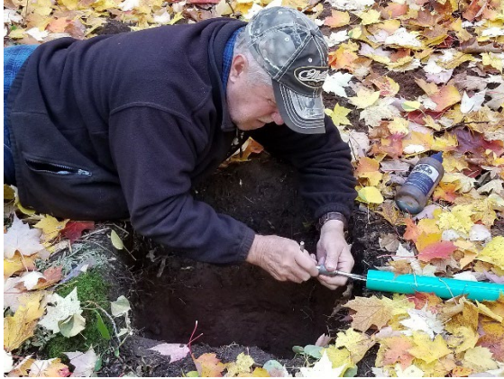
Left: Dennis Karvakko re-tapping threads; Right: getting forms in place to set the equipment in Quikrete
