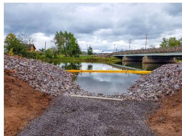
Installing rip rap to protect the notch from erosion
