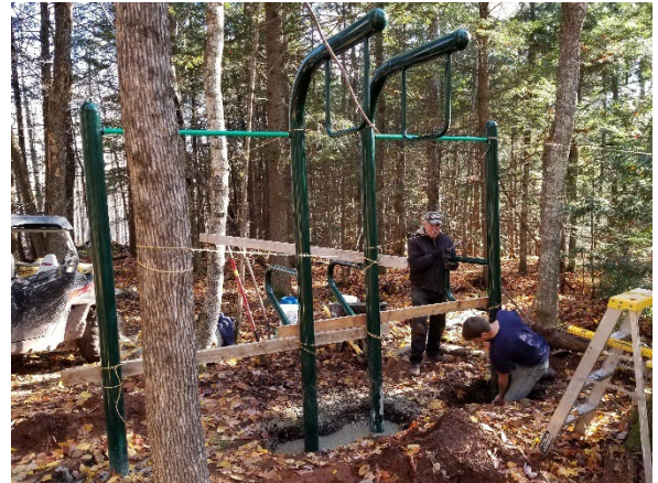
Through a combination of 2 x 4s nailed to trees and twine, Pete found a way to get this station level.
