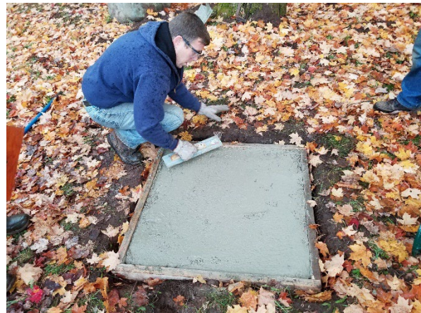
Left: Dan Palosaari and Will Hagelthorn mixing Quikrete; Right: Pete Torola finishing the surface before applying the pattern and adding J-bolts
