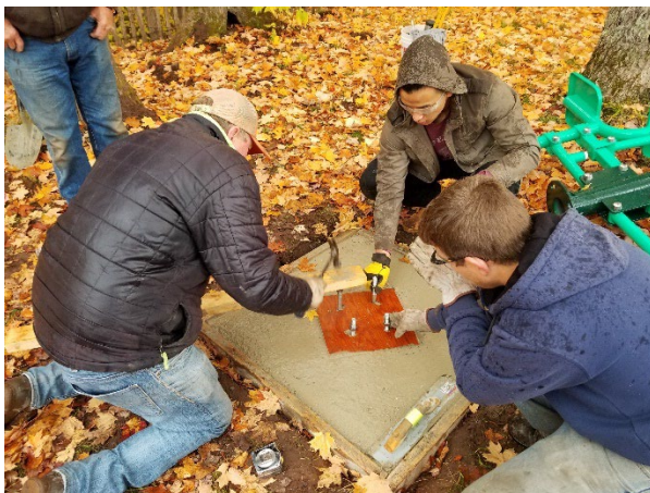
Left: Dan, Will, and Pete setting J-bolts in the pattern; Right: repeating the process for other equipment on the trail held down by J-bolts
