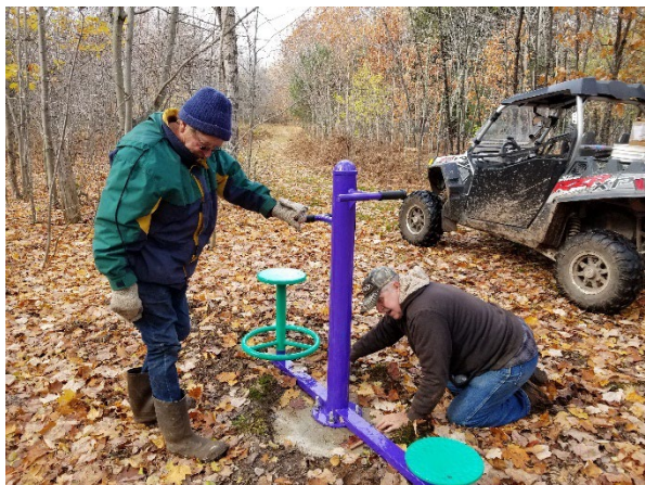
Bill Binroth and Dennis Karvakko tightening down the nuts on the J-bolts
