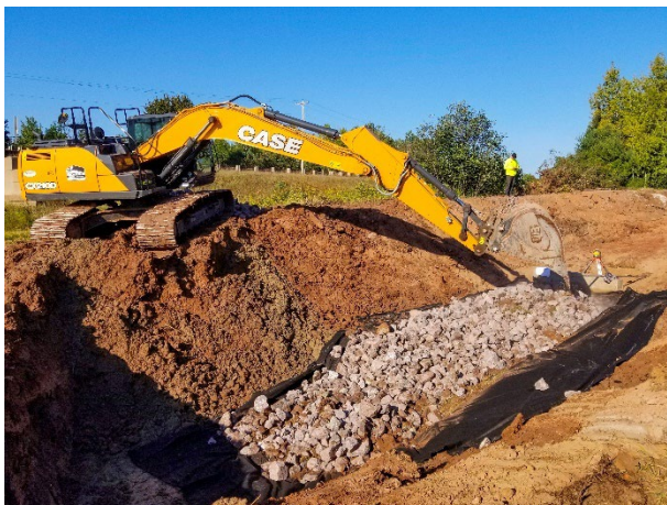
Installing rip rap to protect the notch from erosion
