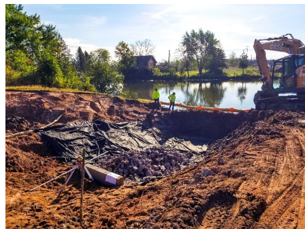
Excavation of the Sturgeon River bank with the headwall already poured.
